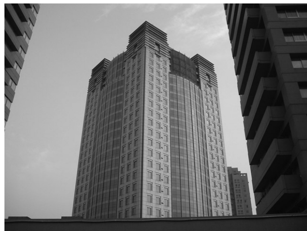
Fig 3. Dashanzi apartment development. (Photo © Ned Rossiter)
