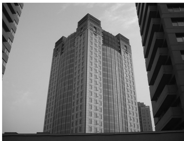
Fig 3. Dashanzi apartment development. (Photo © Ned Rossiter)
